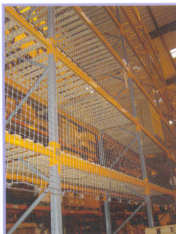
Rear of rack guard
